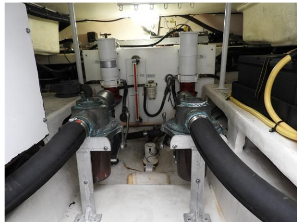
Sea Strainers & Day Tank Looking Aft
