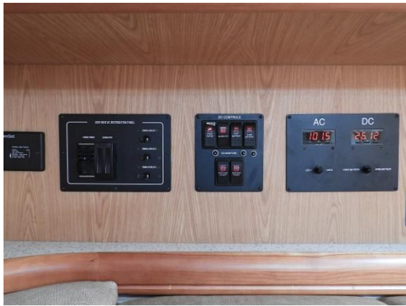
Inside DC Panel
