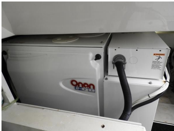
9.5 kw Onan Generator & Soundshield
