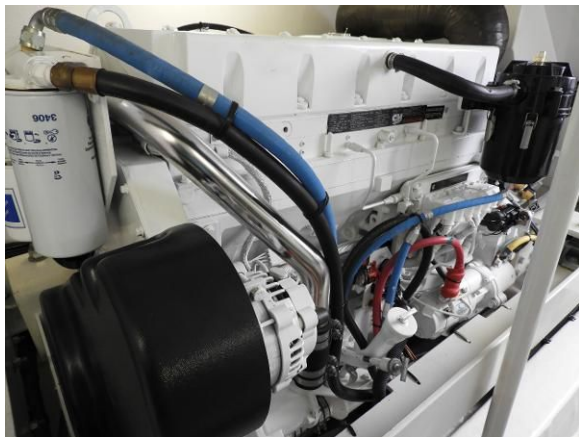
Forward Starboard Engine
