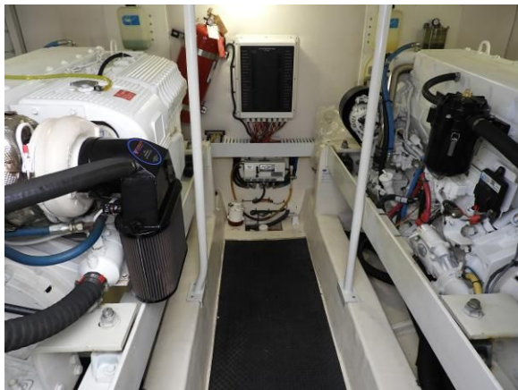
Engine Room looking Forward
