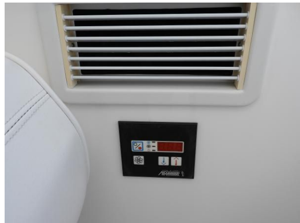
Helm Deck AC Unit
